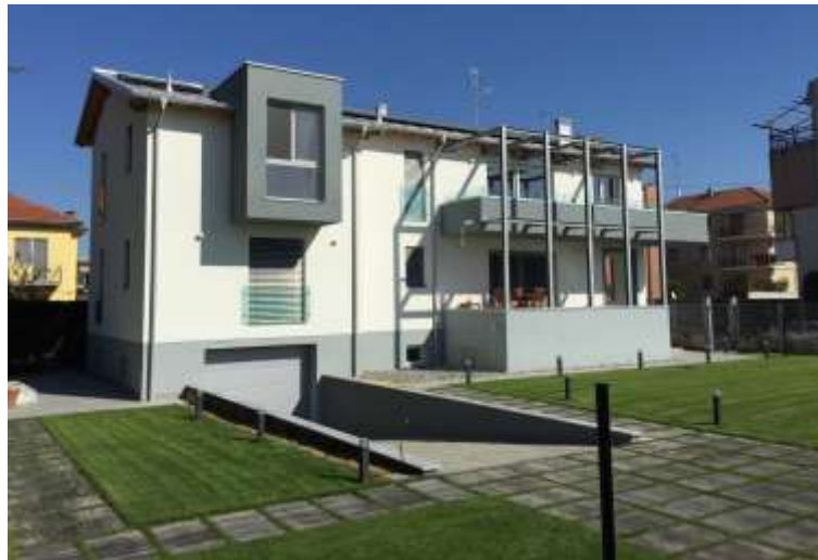
Figure 1. South-facing facade of the reference building.
